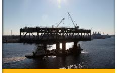
**Gilmerton Bridge span floated into place**
