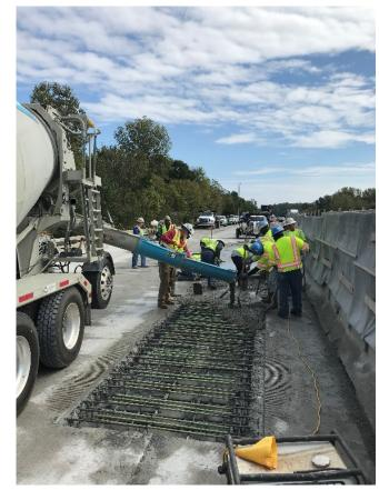
Full depth deck repair (weekend lane closure - hydro concrete demo)
