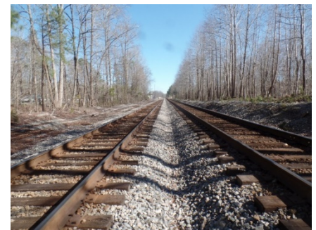
Figure 2: CSXT Railroad Tracks
