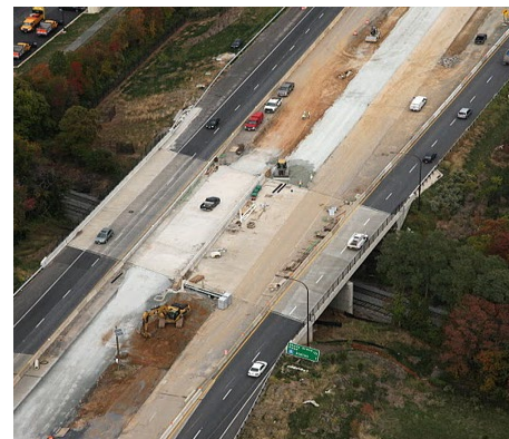
I-370 Bridge over CSXT Railroad
