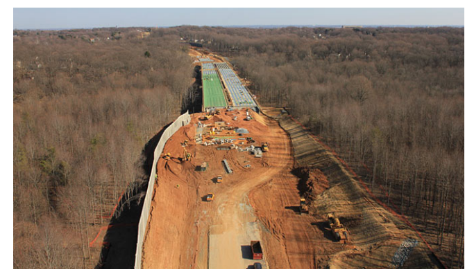
Bridge over Good Hope Stream
