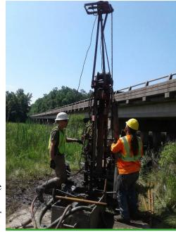
Smaller drill rig used in wetland area to reduce site disturbance.
