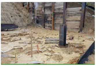
PVD for pre-consolidation, and pipe piles for slope stability and to reduce negative skin friction - I-64 Segment I.
