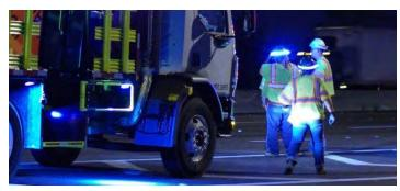
**Figure 3.5-3.** Skanska will explore usage of The Halo Light<sup>TM</sup>, a personal active safety system that attaches to any hard hat and produces a ring of light around the wearer, providing active, 360-degree illumination visible up to ½ mile away. This offers a distinct advantage in being seen by other personnel, motorists, and heavy equipment operators.
