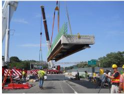
Figure 3.5.4 - Bridge Superstructure Replacement Using Bridge Deck Modules.
