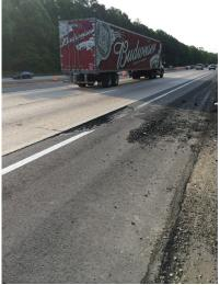
Figure 3.5.5 - Pothole in Strengthened Shoulder
