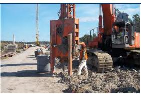
**Geotechnical Mitigation.** Dominion Boulevard's less severe deeper soils were handled by installing 4,400,000 LF of PV (wick) drains and associated drainage layers. Temporary surcharges were installed to accelerate settlement in these areas.
