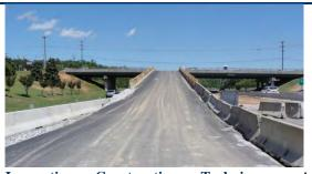
**Innovative Construction Techniques.** A LANE/STV innovative idea involved constructing a median access ramp from a low volume overpass structure to provide construction vehicle access that was SAFELY SEPARATED from highway traffic.
