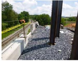
Figure 4: Pile installed after settlement ceased
