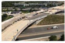
Jones Branch Connector over I-495, Tysons, VA, \$45M – The project involved construction of a new four-lane road and bridge over the I-495 Express Lanes/Jones Branch Drive interchange to Scotts Crossing Road. Improvements were also made along the access road from Jones Branch Drive to the I-495 Express Lanes, and Scotts Crossing Road. A multi-phase TMP was developed and coordination with VDOT and Transurban was critical to the construction over the active interstate and express lanes.
