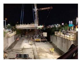
erected at the site using very early strength latex concrete deck closure pours providing the required cure time, strength and durability.
