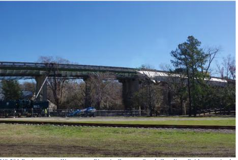
US 501 Business over Waccamaw River in Conway, South Carolina. Bridge required extensive steel repairs, deck joint sealing, concrete crack sealing, spall repairs and a deck hydrodemolition and overlay.
