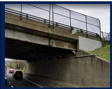
Existing cantilever beams with pin connections used to lengthen the **Broad Street Bridge**. The condition of the anchor bolts in the back of the abutment that hold down the cantilever beams is not known so extreme care will be required when removing the existing deck and superstructure. Temporary modification to this pin connection and the existing restraints may be required to ensure the safety of the traveling public on NB I-95.
