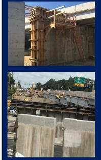
Substructure repair on Rte. 7 bridges over the DTR and DIAAH performed using innovative corrosive protection and specialty concrete allowing for more repairs than VDOT had anticipated while staving within their budget.
