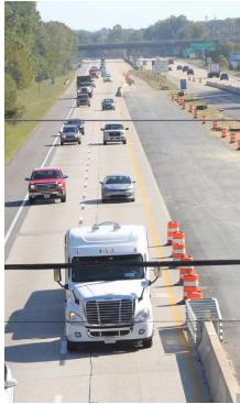
**Figure 3.5.3:**Alternate horizontal alignments can improve ability to maintain full width shoulders during construction, as implemented on I-64.
