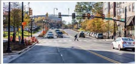
Fort Myer's responsibilities included underground utility installation including dry utility duct banks for Dominion Energy, Verizon, and COMCAST. Roadway improvements included wider sidewalks, curb and gutter, ADA ramps, new street lights, the replacing and/or modifying and upgrading existing traffic signals, and landscaping. A signal light was placed at the intersection of South Frederick Street and Columbia Pike.
