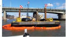
Over-water barge-mounted geotechnical drilling
