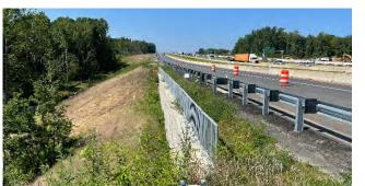
Widening with MSE Wall to eliminate box culvert extension.
