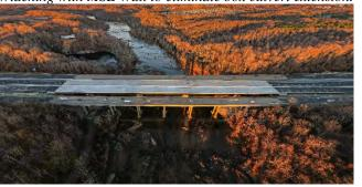
New NB Bridge shifted against the completed SB Bridge.
