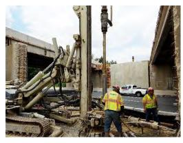
Wagman self-performs all non-disruptive foundations types (such as micro-pile pictured here on Route 7) controlling cost, schedule and reducing work zone requirements.
