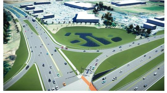
Figure 4.3.1.e-2: Enhanced Extended-Detention Basin in northeast quadrant of the interchange
