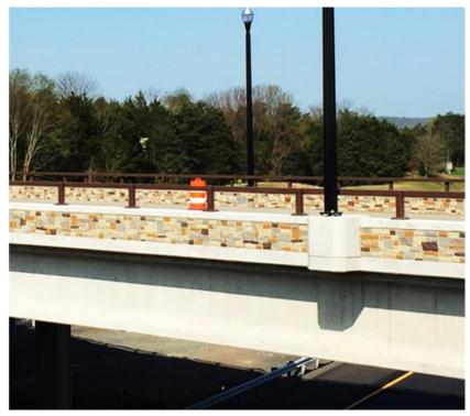
Figure 4.3.2-4 Bridge Parapet with tri-colored Drystack Architectural Treatment: Example from Lane's I-66/Route 15 project.
