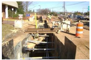
Figure 4.4.2-4: Close coordination with local utility companies (over 30), LANE's \$112M Dulles Metrorail Utility Relocation project mitigated numerous utility impacts and relocations.
