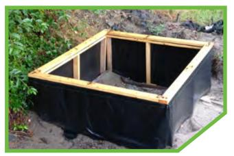
**Figure 4.5.12: Temporary Sediment Traps and Inlet Protection.** We will install similar measures to prevent sediment from entering stormwater conveyance systems prior to permanent stabilization of the disturbed areas.
