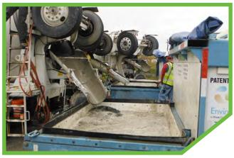
**Figure 4.5.14: Concrete Disposal.** Our crews take appropriate measures to ensure washout water from concrete pours are not released on to the ground or into drains or waterways.
