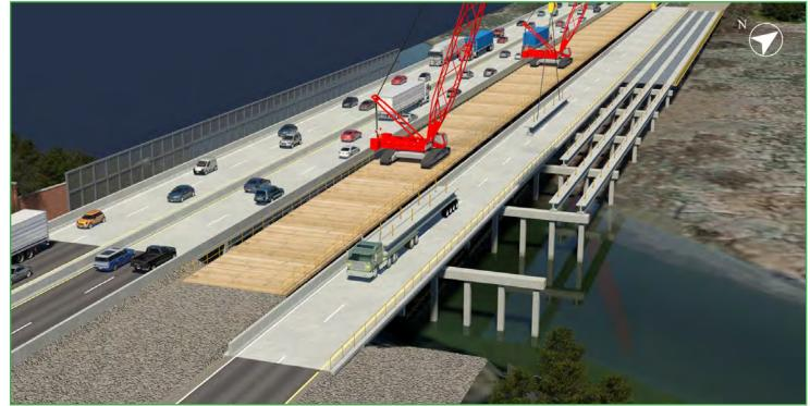
Figure 4.7.15: Install substructure.
