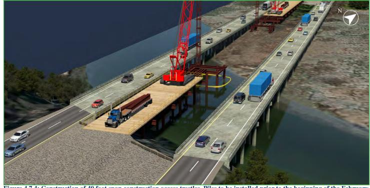
Figure 4.7.4: Construction of 40 foot span construction access trestles. Piles to be installed prior to the beginning of the February Anadromous fish window.
