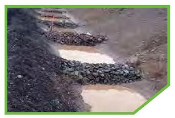
**Figure 4.5.11:Check Dams.** This mitigation measure is effective in small channels with a contributing drainage area similar to those on the I-64 Segment III Project.
