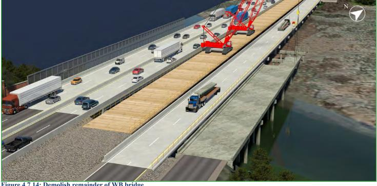
Figure 4.7.14: Demolish remainder of WB bridge.
