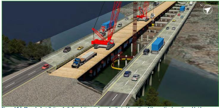
Figure 4.7.5: Phase 1 - Installation of pile foundations and caps for the inside portion of Queens Creek westbound bridge.
