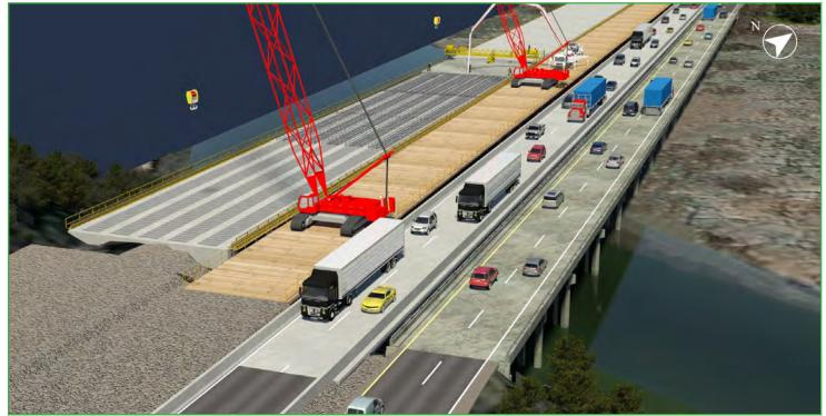
Figure 4.7.12: Pour decks, barrier walls, sound barrier (if required).
