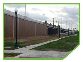
**Figure 4.3.4: Local Experience with Aesthetic Treatments.** Roadway walls completed at I-264 Widening/MLK Extension Project, Portsmouth, VA.
