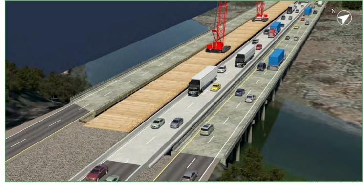
Figure 4.7.8: Install barrier wall on median side and temp barrier on unfinished north side. Hang temporary ITS on median side of WB to maintain camera service. Switch EB traffic onto newly constructed WB using median crossover. Enter Phase 2.
