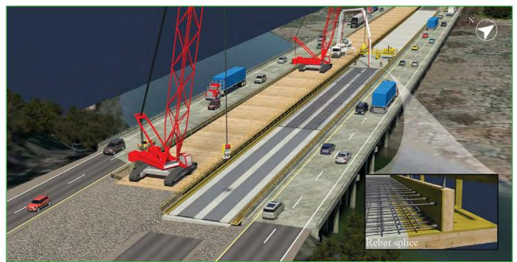
Figure 4.7.7: Install stay in place deck forms stainless deck reinforcing steel (rebar splice detail shown for construction of WB widening in Phase 3).
