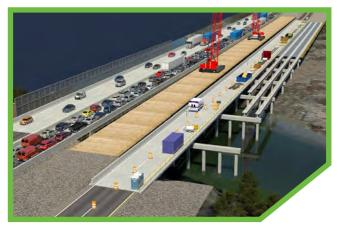
**Figure 4.5.18: Queens Creek Bridge Phase 3:** Our crews will maintain a delineated access lane for emergency responders to use during hours that our crews are not present in Phase III of the Queens Creek Bridge construction.
