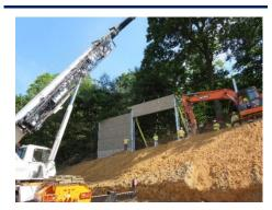
Figure 4.5.1-6. LANE's I-66 WB (Spot Improvements project) also included noise barrier installation.
