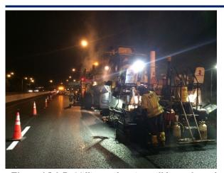
Figure 4.5.1-7. Milling and paving will be performed overnight to minimize impacts to the traveling public.
