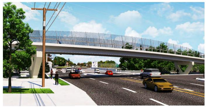
Hiking & Biking Trail No. 4 over I-66 (B-681). Modifications to this Hiking & Biking Trail Bridge include the relocation of Pier 3 to accommodate the widening of I-66 EB. The new pier is anticipated to consist of 2 drilled shafts located laterally outside of the footprint of the existing pier to avoid conflicts with the existing footing. The existing superstructure will be analyzed and strengthened/modified
