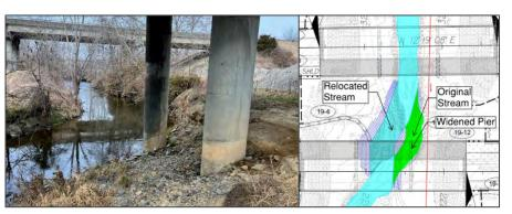
Figure 4.3.2-5: Lewis Creek Existing ScouredFigure 4.3.2-6: Relocated Lewis<br/>ConditionConditionCreek
