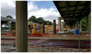
Figure 4.4.7 Bridge Widening Near Railroad with Soft and Loose Subsurface Soils that our Lead Geotechnical Engineer Worked on
