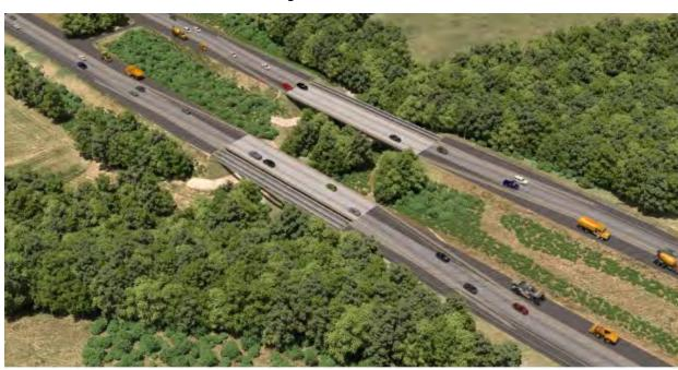
Roadway remains shifted to the right; traffic on bridges is shifted to the left; traffic shifts are required between roadway and bridges
