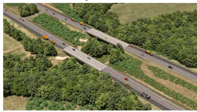
Roadway and bridges are one lane; no traffic shifts required between roadway and bridge
