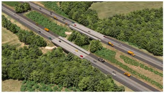
Roadway and bridges are two lanes but are shifted to the right; traffic shifts are required between roadway and bridges
