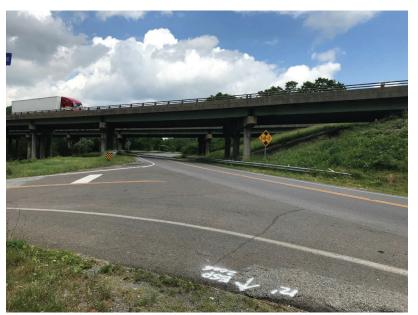
Figure 4.3.1(a): Route 11 Existing Conditions to Remain - Proposed Clearance to be 16'-6" Min.
