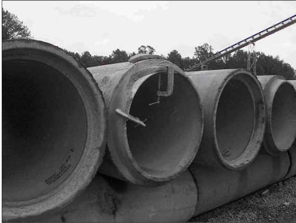
Photo 26 - Pipe with Formwork
