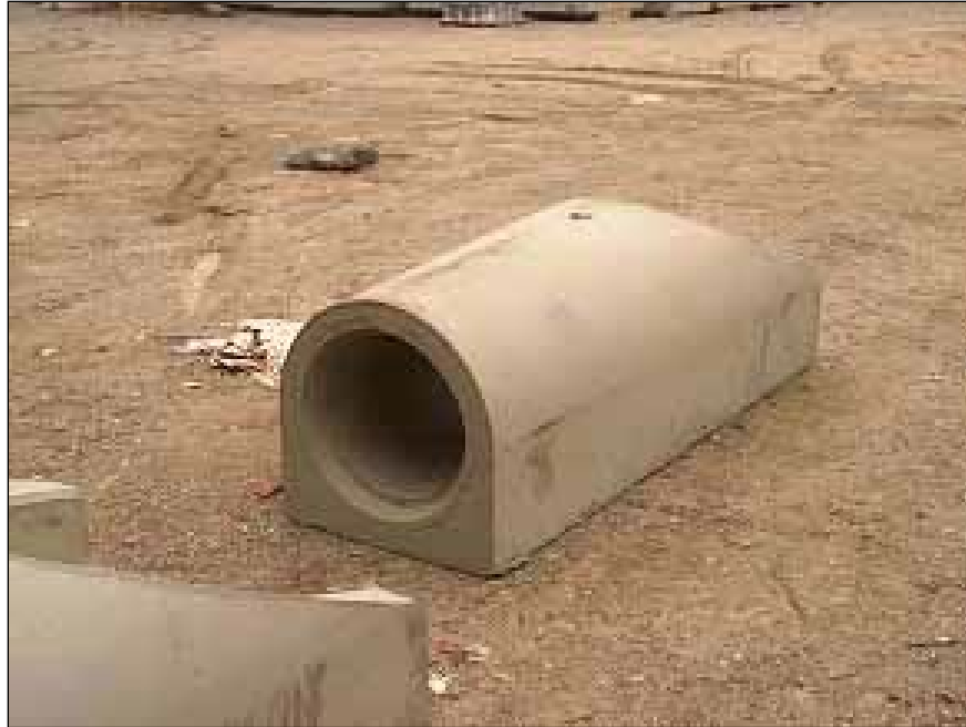
Photo 18 - Grooved Flared End Section
