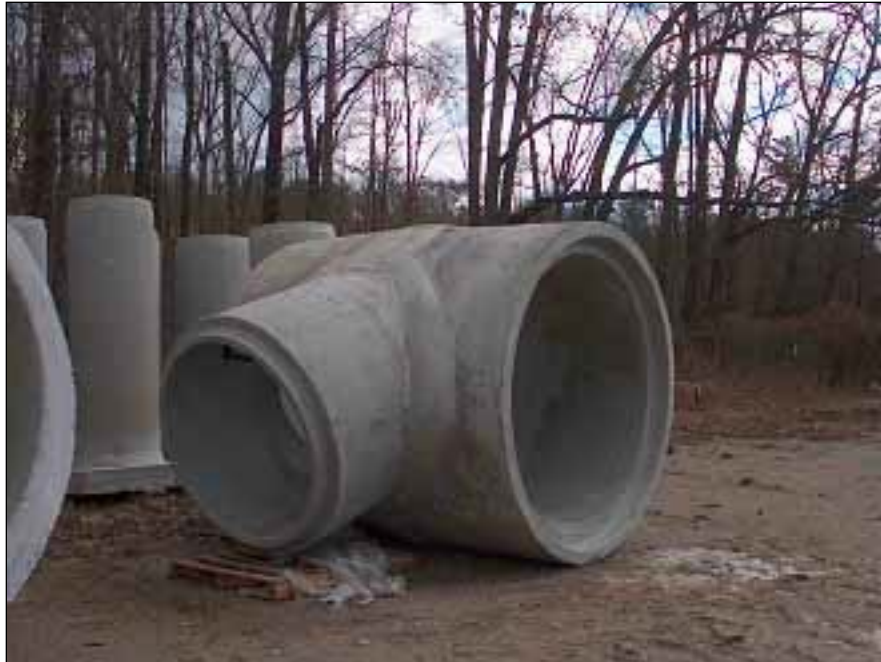
Photo 16 - Manhole Tee Base
