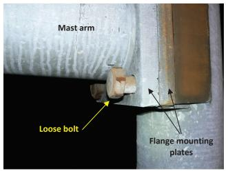
**Photo 5.55** Loose bolt at flange mounting plates of mast arm to pole connection
