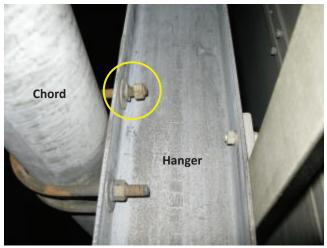
Photo 4.78 Loose nut on hanger to chord U-bolt
