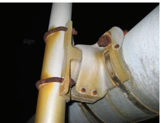
Photo 5.85 Corrosion on non-stainless connection hardware of orbital bracket
