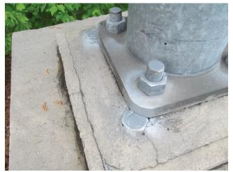
Photo 5.35 New pole/base plate connected to previous baseplate which is buried in grout
