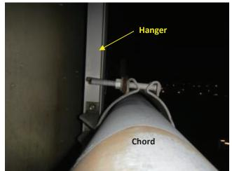
**Photo 4.84** Oversized clamp at hanger to chord connection of double arm trussed sign
