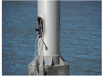
Photo 6.43 Missing hand hole cover with wires exposed
