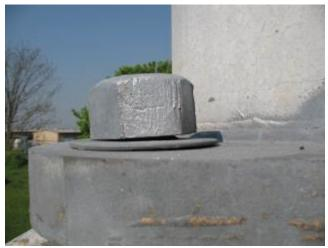
Photo 4.25 Top nut improperly seated on base plate
