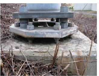
Photo 6.51 8-bolt pedestal to 4-bolt pole extension retrofit
