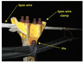
**Photo 5.90** Moderate corrosion on span wire clamp bolts and pin at leveling assembly connection
