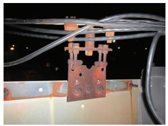
Photo 5.92 Corrosion and wear on sign attachment hardware
