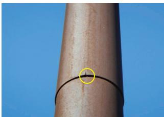
Photo 6.40 Crack at slip joint
