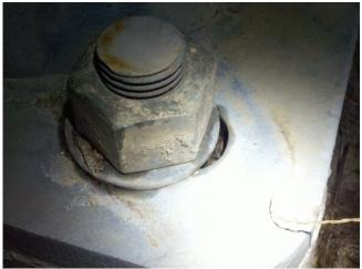
**Photo 5.32** Oversized hole in base plate and Inadequately sized flat washer under top nut
