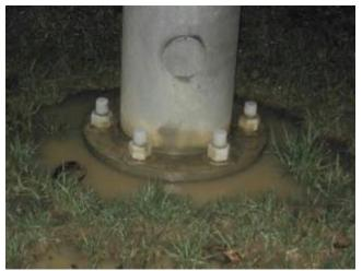
**Photo 4.10** Standing water around base of pole located in swale/drainage ditch
