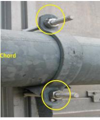
**Photo 4.75** Missing flat washers at hanger to chord connection. Lock washers too small for slotted holes.
