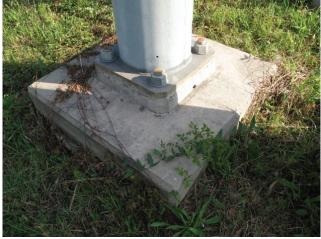
Photo 5.24 Sound grout pad with weep hole
