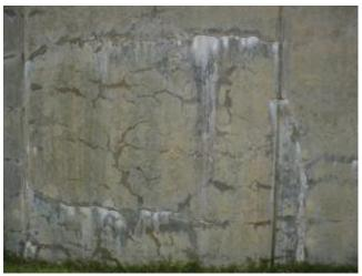
Photo 3.3 Map cracking with efflorescence
