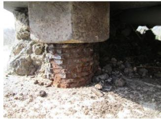
Photo 5.26 Heavy corrosion and section loss on anchor bolt below leveling nut
