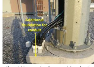
Photo 1.83 Trussed Cell tower with multiple foundations
