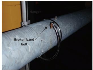
*Photo 5.88* 1 of 2 broken band bolts on orbital bracket
