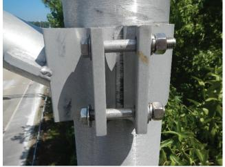
Photo 6.56 Loose chord collar connection bolt
