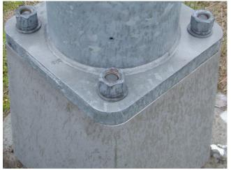
Photo 6.23 Top nuts less than 100% engaged
