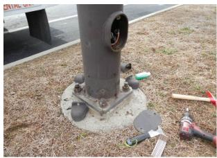
Photo 6.39 Corrosion of base plate
