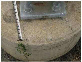
Photo 6.14 Cracks in pedestal extending out from anchor bolts
