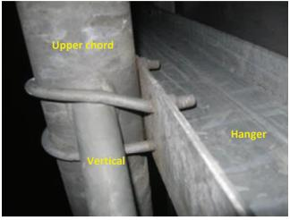
Photo 4.81 Misaligned and bent U-bolt at hanger to chord connection
