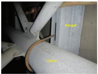
Photo 4.80 Missing nut on hanger to chord connection Ubolt
