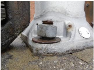
Photo 6.26 Out of plumb anchor bolt and loose top nut
