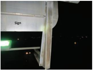
Photo 4.76 Bent/Twisted hanger from impact damage
