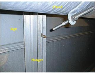
**Photo 4.82** Broken hanger to chord attachment of extruded sign panel
