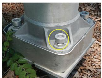
Photo 6.35 Torque control component installed upside down and not separated from nuts
