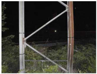
Photo 4.37 Bowed/Bent pole (I-beam)
