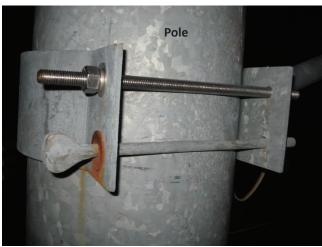
Photo 5.49 Corroded sign to pole connection hardware
