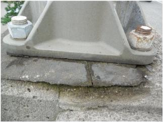
*Photo 6.20 Deteriorated grout pad with moisture leakage*
