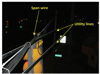
**Photo 5.74** Span wire resting on top of utility lines
