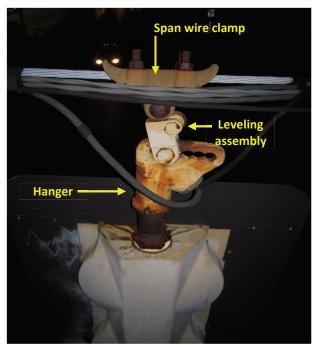
Photo 1.53 Leveling pipe assembly
