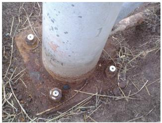
Photo 4.33 Corrosion and section loss on base plate
