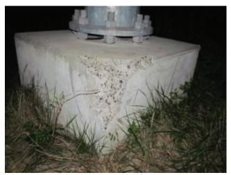
Photo 3.1 Spall due to impact damage
