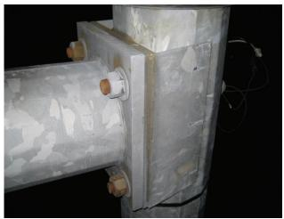
Photo 1.31 Gusseted box flange connection
