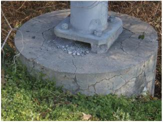
Photo 6.19 Deteriorated grout pad
