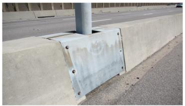
Photo 2.10 Ancillary structure in barrier with barrier plates
