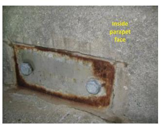
**Photo 4.66** Corrosion and minor pitting on through bolt parapet attachment plate (traffic side of parapet)
