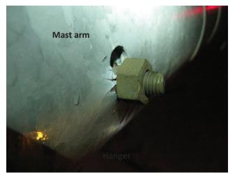
Photo 5.68 Tear in bolt hole in mast arm at bolted slip joint
