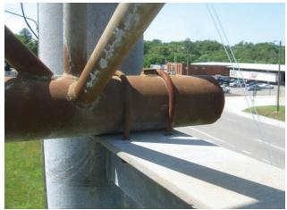
Photo 1.13 Simple truss support, seated on strut of vertical support
