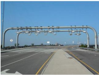
Photo 1.9 Overhead span, monotube structure
