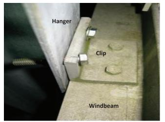
**Photo 4.77** Crack in aluminum angle clip at windbeam to hanger connection
