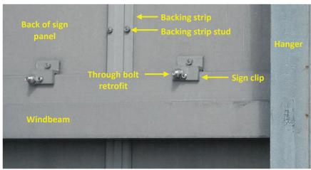
Photo 1.3 Sign panel attachment to windbeam with retrofitted through bolt
