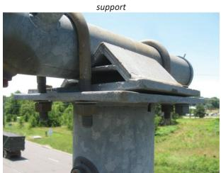
Photo 1.15 Simple truss support, seated on pole
