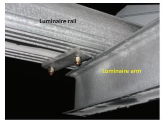
**Photo 4.101** Loose luminaire rail clip at rail to luminaire arm connection
