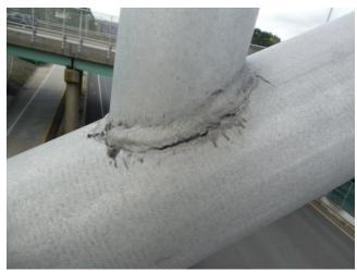
Photo 6.63 Lower chord member to strut weld cracked
