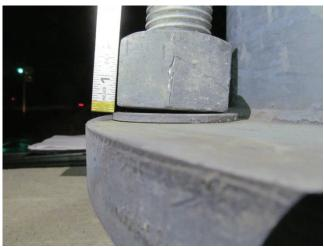
Photo 5.28 Top nut improperly seated on base plate
