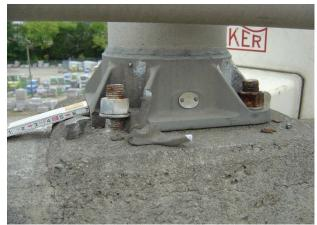
Photo 6.38 Broken base plate at anchor bolt
