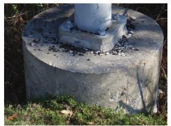
Photo 6.8 Map cracking with efflorescence in pedestal
