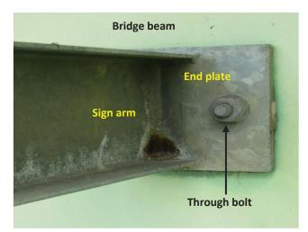
Photo 1.41 Attachment to bridge beam, through bolt
