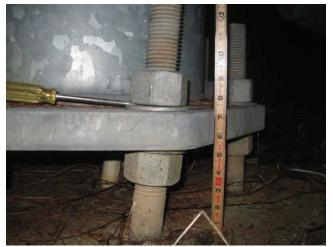
Photo 4.28 Out of plumb anchor bolt
