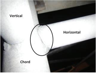
Photo 4.54 Broken weld at horizontal truss to chord connection
