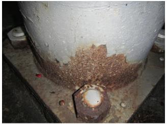
Photo 5.34 Corrosion and pitting on base plate, bottom of pole and on anchor bolt and top nut
