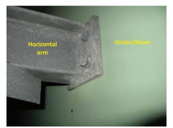
**Photo 4.67** Loose bolt at lower horizontal arm to girder/beam connection
