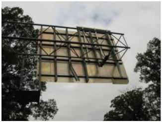
Photo 4.69 Impact damage to hangers and windbeams
