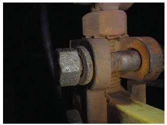
Photo 5.93 Loose bolt at hanger assembly on signal attachment to span wire
