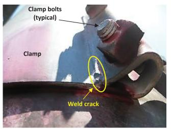
**Photo 4.71** Weld crack (verified with dye penetrant)in hanger to chord connection clamp (two chord truss)
