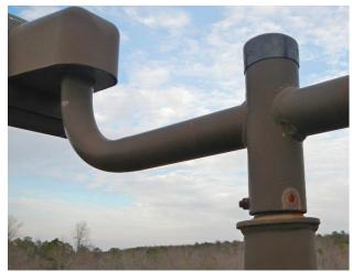
Photo 6.64 Sheared tenon set screw with corrosion
