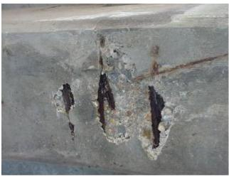
Photo 3.4 Spalling with exposed reinforcing steel
