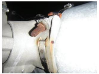
**Photo 3.36** Galvanic corrosion of strap bolt and zinc strap pin due to stainless steel strap, nut and washer
