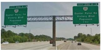
Photo 1.34 Butterfly, four chord box truss
