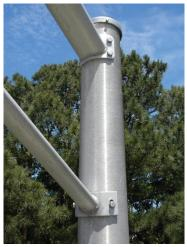
Photo 6.6 View of chord to pole connection
