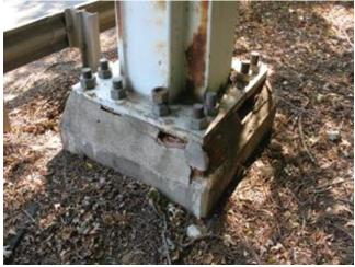
Photo 4.20 Partially deteriorated grout pad
