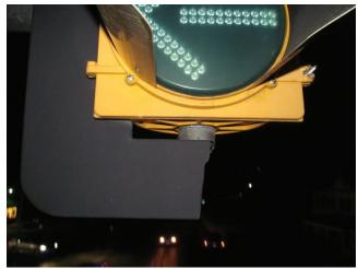
Photo 5.96 Broken backplate on signal head
