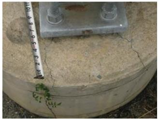
Photo 4.14 Cracks in pedestal extending out from anchor bolts
