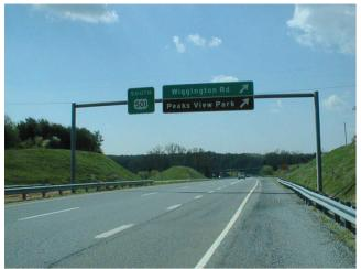
Photo 1.8 Overhead span, single chord and pole structure
