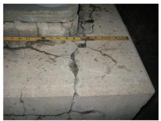
Photo 5.10 Map cracking in pedestal
