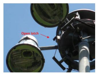
Photo 6.65 Open latch on luminaire ring
