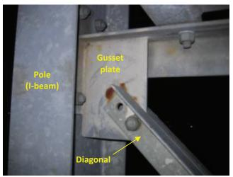
Photo 4.44 Missing bolt at diagonal member to gusset plate connection on pole (I-beam)
