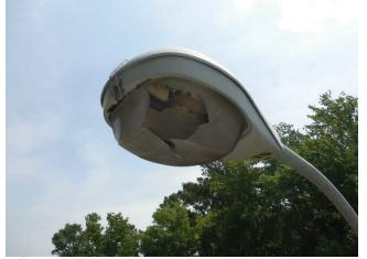
Photo 6.67 Luminaire head lens broken
