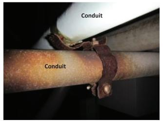
**Photo 4.94** Heavily corroded and broken conduit straps
