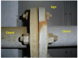
**Photo 4.56** Gap in of upper half of upper chord splice flanges and breakdown of galvanizing (brown color) with light corrosion
