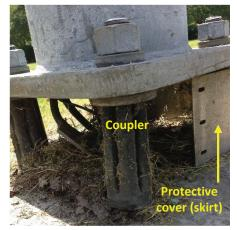
Photo 1.67 Cast aluminum breakaway coupler
