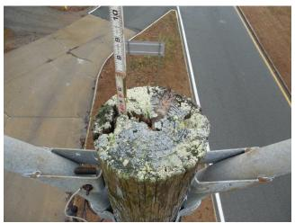
Photo 6.53 Timber pole decay and splitting
