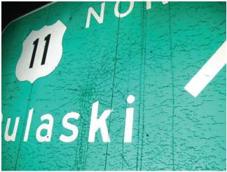
**Photo 4.91** Crazing/cracking of sign panel reflective material
