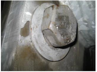
**Photo 5.57** Oversized flat washer under bolt at flange mounting plates of mast arm to pole connection
