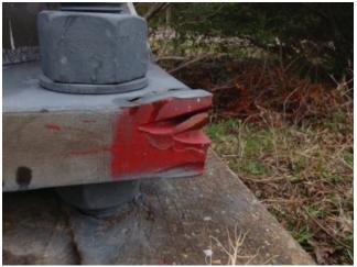
Photo 5.33 Impact damage to base plate
