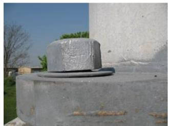
Photo 6.24 Top nut not fully seated on base plate
