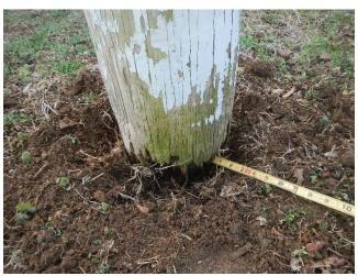
Photo 6.52 Timber pole decay below grade
