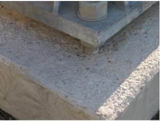
Photo 6.13 Scaling on top of pedestal
