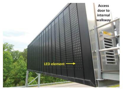
Photo 1.6 VMS panel, LED type with internal walkway
