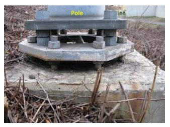
Photo 4.45 8-bolt pedestal to 4-bolt pole extension retrofit
