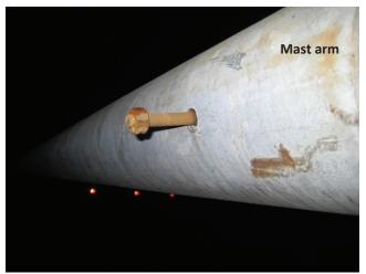
**Photo 5.67** Loose, oversized (length), and undersized (diameter) bolt at bolted mast arm slip joint
