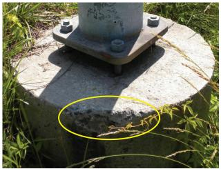
Photo 6.9 Spall in pedestal
