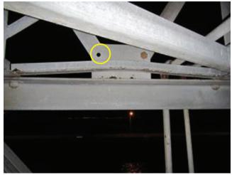
**Photo 4.58** Missing diagonal truss bolt at chord panel point and bent horizontal truss
