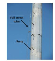
Photo 1.80 Integrated rungs and fall arrest system
