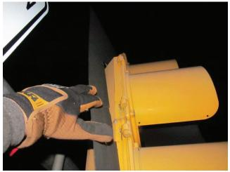
Photo 5.97 Detached backplate on signal head
