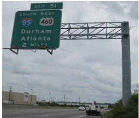
Photo 1.30 Cantilever, four chord space truss
