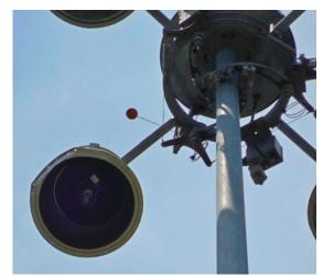
Photo 6.66 Missing luminaire lens on luminaire ring
