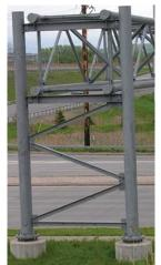
Photo 1.23 Two pole truss (end frame)
