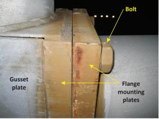
**Photo 5.60** Loss of galvanization and light corrosion on flange mounting plates, bolts and washers at mast arm to pole connection
