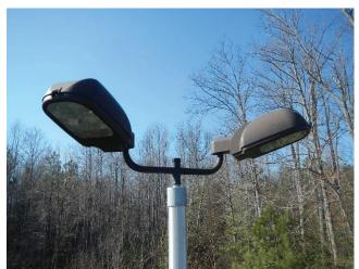
Photo 6.5 View of offset luminaire heads
