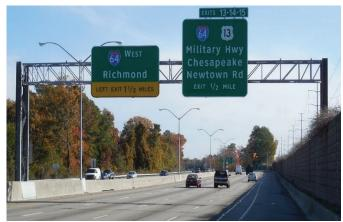
Photo 1.24 Overhead span with barrier mount foundation
