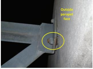
Photo 4.65 Pull out of anchor bolt at sign attachment to parapet
