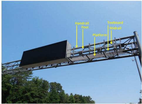
Photo 1.7 Overhead span with walkway
