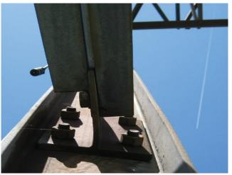
Photo 1.19 Bolted T-shape connection
