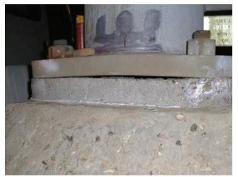
Photo 4.32 Distorted/bowed base plate
