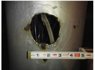
Photo 5.41 Torch cut hole in pole
