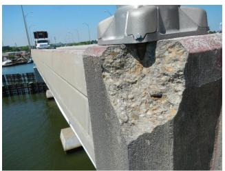
Photo 6.15 Spall in bridge parapet
