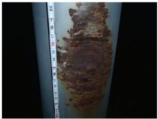
**Photo 5.42** Impact damage to painted pole with corrosion on affected area
