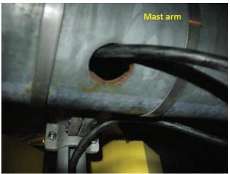
**Photo 5.69** Corrosion around electrical port and missing rubber grommet
