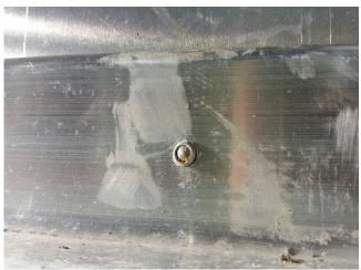
**Photo 4.89** Loose through rivet at sign panel to windbeam connection
