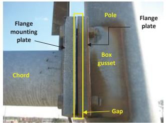
**Photo 4.49** Gap in flange mounting plates of chord to pole connection
