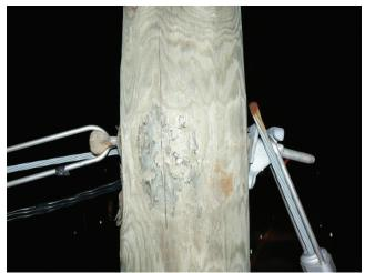
**Photo 5.63** Bent thimble eye bolt on timber pole due to guy wire attached on backside of bolt
