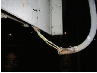
Photo 4.95 Broken conduit with exposed wiring
