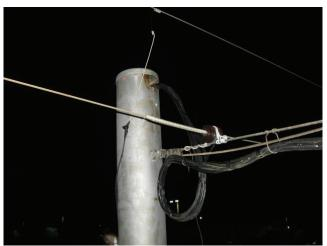
Photo 5.9 View of span wire to pole connection
