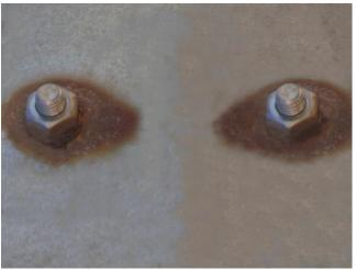
**Photo 3.38** Localized galvanic corrosion of galvanized steel plate due to stainless steel bolts
