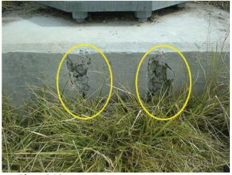
**Photo 6.16** Areas of poor consolidation in pedestal (Sign structure shown for illustrative purposes only)
