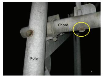
*Photo 4.61 Missing cap on chord electrical port*
