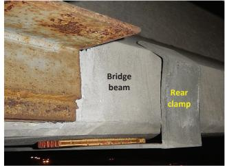
**Photo 1.43** Attachment to bridge beam, saddle clamp, rear view
