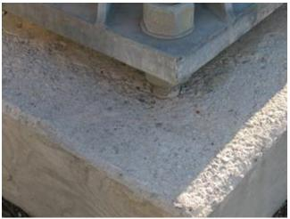
Photo 4.13 Scaling on top of pedestal
