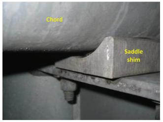
Photo 4.51 Undersized saddle shim at chord to pole connection
