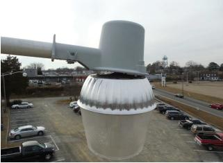
Photo 6.68 Luminaire head loose
