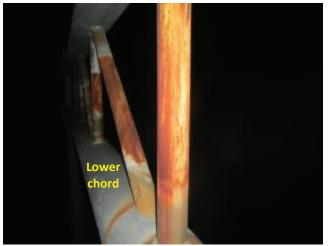
Photo 4.60 Light corrosion on chord trussing
