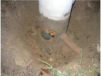
**Photo 4.47** Buried pole and horizontal truss with heavy corrosion and section loss
