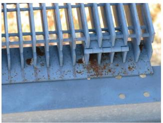
**Photo 4.93** Corrosion on walkway grating support beam and around grating hinge
