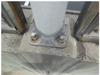
**Photo 6.27** Oversized hole in base plate and inadequately sized flat washer under top nut
