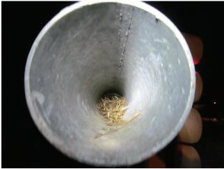
Photo 5.73 Missing end cap on mast arm with bird nesting debris inside arm
