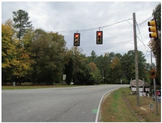
**Photo 5.2** Front view of structure with span wire governing single travel direction
