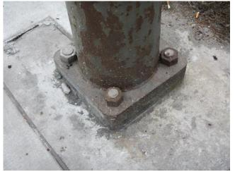
**Photo 5.20** Foundation adjacent/level with concrete sidewalk, corrosion on base plate, pole, and top nuts.
