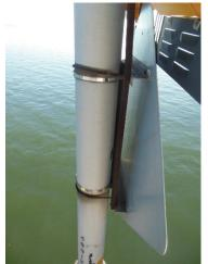
Photo 6.55 Corroded sign to pole connection hardware
