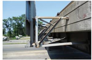
Photo 1.38 Bridge parapet mount sign, side view
