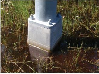
**Photo 6.10** Standing water around transformer base located in a swale/drainage ditch
