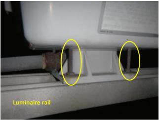
**Photo 4.99** Corroded luminaire housing to luminaire track attachment bolts
