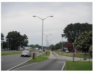
**Photo 2.12** Conventional luminaires over the scales at a weigh station
