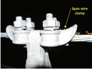
Photo 5.91 Loose bolts at span wire clamp
