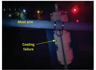
**Photo 5.95** Misaligned signal head, note coating failure on backside of signal head
