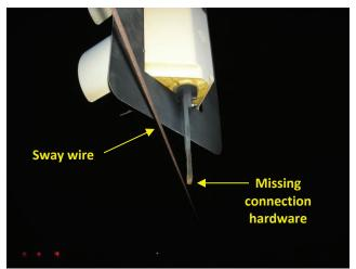
**Photo 5.94** Missing connection hardware at signal head to sway wire connection
