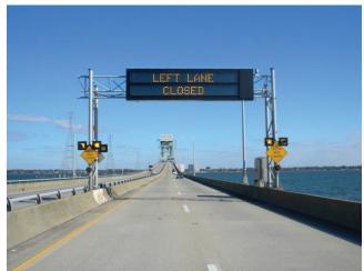
Photo 1.2 Overhead span sign structure
