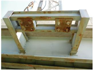
Photo 4.18 Corrosion of steel haunch
