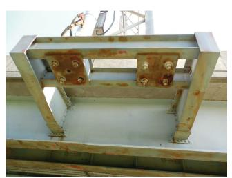
**Photo 6.18** Corrosion of steel haunch (Sign structure shown for illustrative purposes only)
