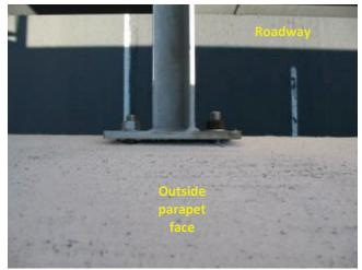
**Photo 4.64** Gap between mounting plate and parapet at sign attachment to parapet
