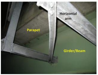
Photo 4.68 Bent horizontal diagonal
