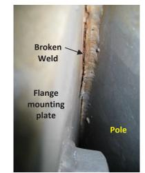
Photo 5.56 Broken weld at flange mounting plate to pole connection
