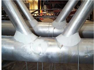
Photo 3.41 Fiber reinforced plastic repairs to sign structure
