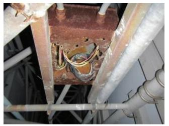
**Photo 4.96** Heavy corrosion and section loss on junction box with exposed wiring
