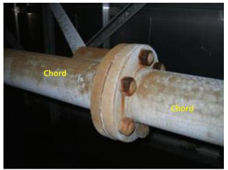
**Photo 4.55** Loss/Breakdown of galvanizing with corrosion of the chord, splice plates, and splice bolt nuts
