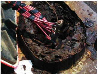
**Photo 3.30** Corrosion and section loss/break at base of high mast light
