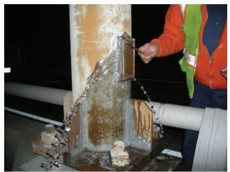
Photo 6.42 Pole holding water, released on loosening of hand hole cover
