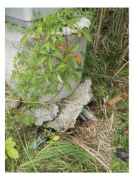
Photo 6.12 Overgrowth of vegetation on, and erosion of, pedestal
