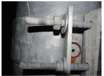
Photo 5.51 Loose nut at luminaire attachment saddle clamp
