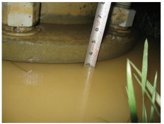
**Photo 5.12** Standing water around base of pole located in a swale/drainage ditch
