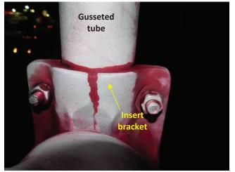
Photo 5.81 Crack in insert bracket at gusseted tube connection on orbital bracket
