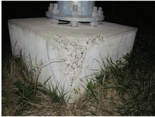
Photo 5.11 Spall in pedestal
