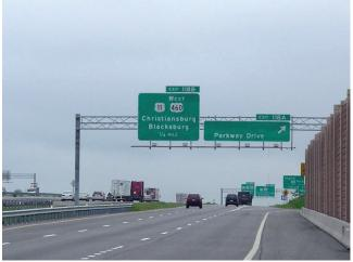
**Photo 2.11** Sign structure with right pole behind a sound wall
