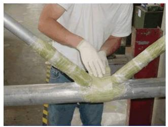
**Photo 3.40** Application of fiberglass repairs to sign structure
