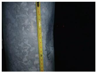
Photo 5.43 Impact damage/dent to pole
