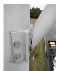
Photo 6.60 Lower chord to pole connection cracked/broken
