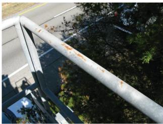
Photo 4.92 Localized corrosion on walkway handrail
