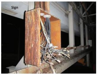
Photo 4.98 Open junction box with exposed wiring
