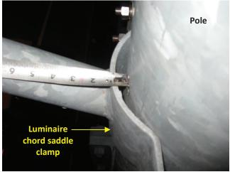
Photo 5.50 Undersized luminaire attachment saddle clamp
