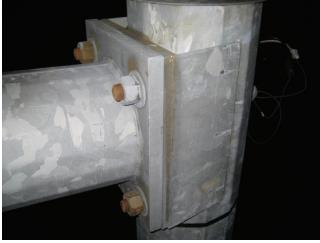
Photo 1.16 Gusseted box flange connection
