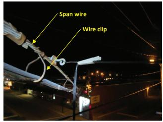
**Photo 5.75** Loss of galvanization on span wire and wire clips with light to moderate corrosion
