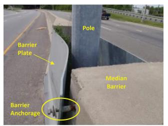
**Photo 6.17** Damaged median barrier plate with failed/pulled out barrier anchorage
