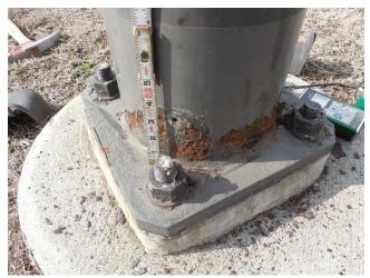
Photo 6.50 Corrosion at base of pole
