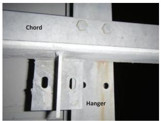
Photo 4.74 Misaligned hanger to chord connection
