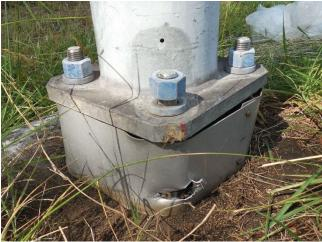
Photo 6.31 Protective skirt damaged and top nut loose
