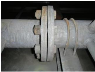
Photo 4.62 Gap in lower half of upper chord splice
