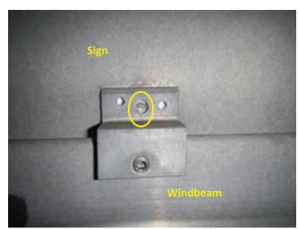
Photo 4.85 Loose through bolt of sign to windbeam connection
