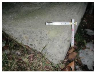
Photo 4.9 Spall in pedestal
