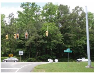
**Photo 5.6** Secondary view of span wire governing two routes
