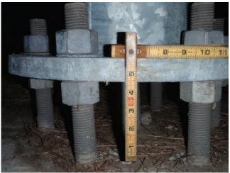
Photo 5.29 Loose leveling nut and missing flat washer
