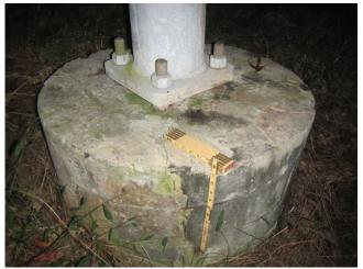
**Photo 5.16** Crack in pedestal extending out from anchor bolt
