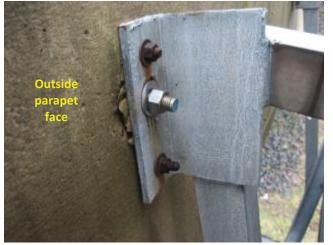
Photo 4.63 Spalling behind sign attachment to parapet
