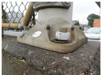
Photo 6.21 Loose top nut and bent anchor bolt
