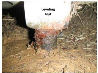
Photo 4.23 Heavy corrosion and section loss on anchor bolt below leveling nut
