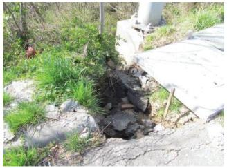
Photo 5.17 Erosion around back side of pedestal
