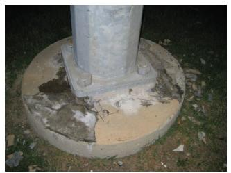
Photo 5.15 Delamination on top of pedestal
