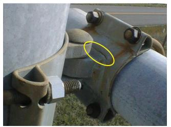
Photo 4.52 Cracked weld at single chord to pole connection
