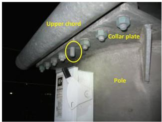
**Photo 4.50** Missing nut on collar plate bolt at upper chord to pole connection
