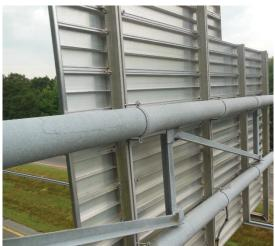
Photo 1.4 Sign panel, extruded type, rear view
