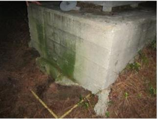
**Photo 4.15** Erosion and undermining around back side of pedestal
