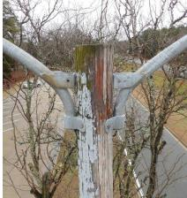
Photo 1.64 Luminaire arm to timber pole connection, through bolted
