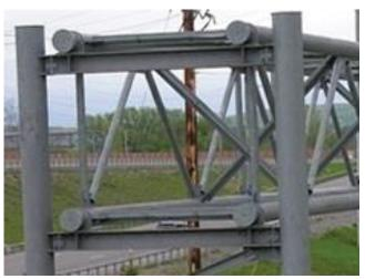
Photo 4.6 View of chord to pole connection
