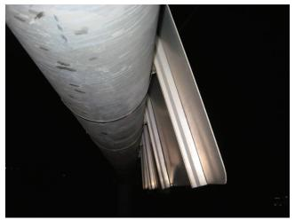
Photo 5.101 Impact damage to sign mounted to mast arm
