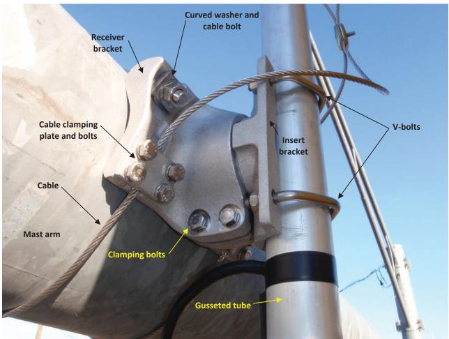
Photo 5.77 Typical cable mount orbital bracket
