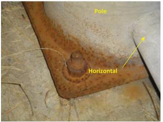
Photo 4.41 Light corrosion of base plate to pole weld
