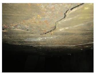
Photo 3.6 Delamination and spalling
