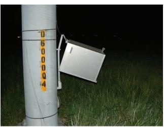
Photo 5.52 Failed securing straps on control box mounted to pole
