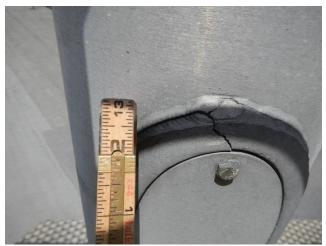
Photo 6.49 Crack in weld at hand hole cover
