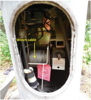
Photo 1.74 High mast light pole hand hole
