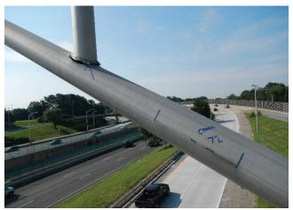
**Photo 6.61** Lower chord member and weld along strut cracked
