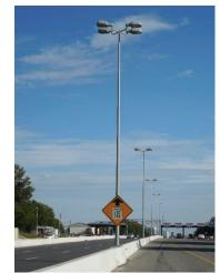
Photo 1.70 Offset luminaire, quad mount
