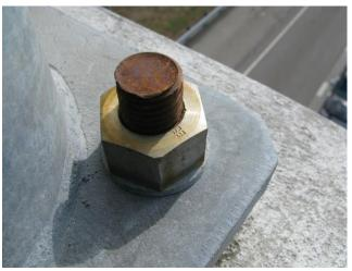
Photo 3.37 Galvanic corrosion of galvanized steel anchor rod to stainless steel nut
