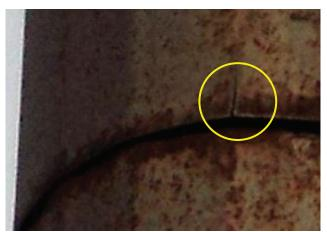
Photo 6.41 Crack at slip joint
