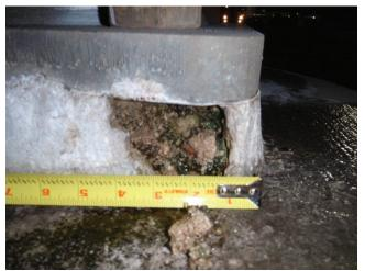
Photo 5.22 Partially deteriorated grout pad with moisture leakage
