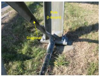
Photo 4.42 Impact damage to pole trussing diagonal
