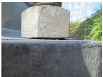
Photo 5.25 Loose top nut and missing flat washer
