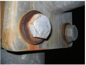
**Photo 5.58** Corrosion on excessive flat washers at flange mounting plates of mast arm to pole connection
