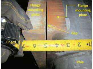
**Photo 5.53** Gap in flange mounting plates of mast arm to pole connection
