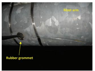
Photo 5.70 Impact damage to mast arm
