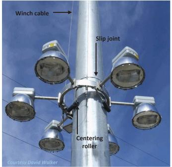
Photo 1.73 High mast light luminaire ring being lowered
