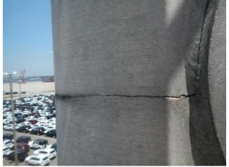
**Photo 6.48** Crack in weld at hand hole cover extending into pole
