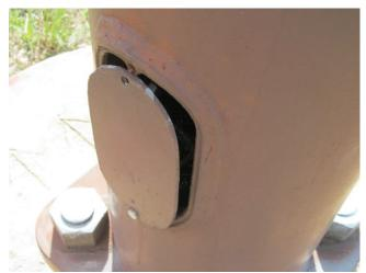
Photo 5.36 Loose hand hole cover due to sheared top bolt
