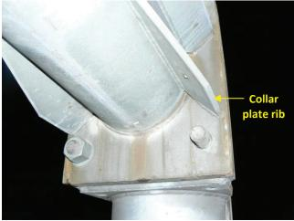
**Photo 5.54** Missing nut on flange mounting plate of mast arm to pole connection
