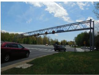
Photo 1.56 Overhead span, single chord, traffic signal
