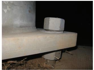
Photo 5.31 Out of plumb anchor bolt with improperly seated top nut
