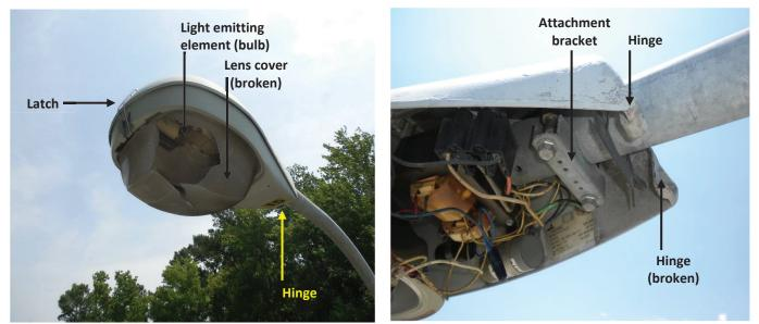
Photo 1.60 Luminaire housing exterior
