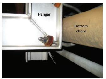
**Photo 4.73** Oversized U-bolts with dissimilar metals (stainless steel U-bolt with mild steel washers) and excess washers at hanger to chord connection
