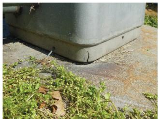
**Photo 6.33** Transformer base with crack at bottom adjacent to anchor bolt
