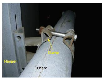
**Photo 4.72** Dissimilar metals (stainless steel bolt and galvanized clamp) at hanger to chord connection clamp (two chord truss)
