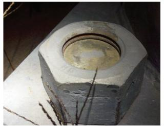
Photo 5.27 Top nut 75% engaged and missing flat washer
