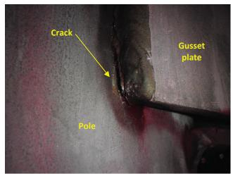
Photo 5.59 Crack in weld at gusset plate at mast arm to pole connection
