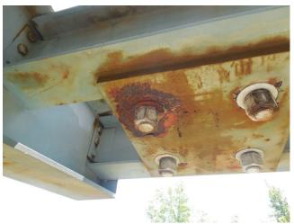
**Photo 4.19** Coating failure and corrosion on steel haunch members and connection hardware
