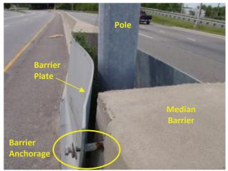
**Photo 4.17** Damaged median barrier plate with failed/pulled out barrier anchorage (Luminaire structure shown for illustrative purposes only)
