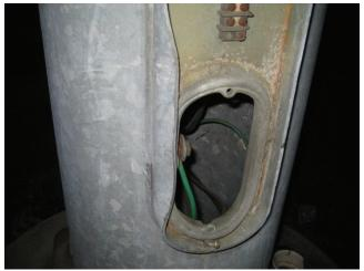
Photo 5.37 Missing hand hole cover, bent ring around hand hole
