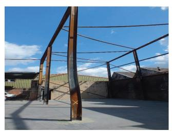
Photo 3.21 Fire damage and out of plane distortion
