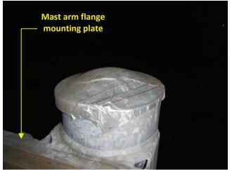
**Photo 5.39** Broken pole cap with duct tape in place over missing portion of cap
