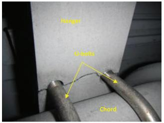
**Photo 4.79** Cracked hanger at hanger to chord connection U-bolt
