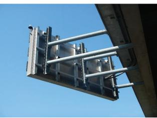
Photo 1.40 Bridge parapet mount VMS, rear view
