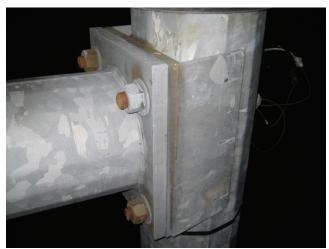
Photo 5.8 View of mast arm to pole connection
