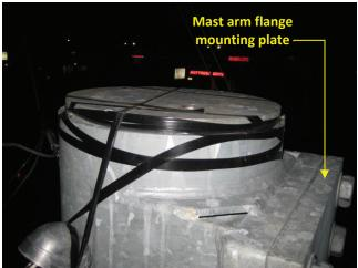
Photo 5.38 Loose pole cap secured with electrical tape
