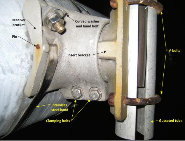
Photo 5.76 Typical band mount orbital bracket
