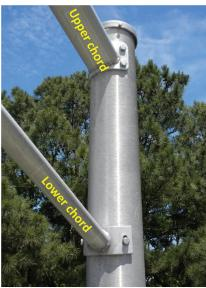
Photo 1.62 Luminaire arm to pole connection, bolted
