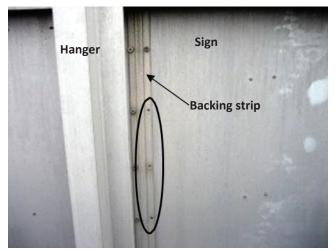
Photo 4.87 Sheared backing strip studs
