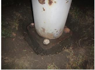
**Photo 5.44** Buried base plate with corrosion and pitting on base plate, base plate to pole weld and pole
