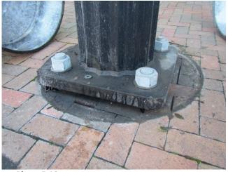
Photo 5.18 Foundation located under brick sidewalk
