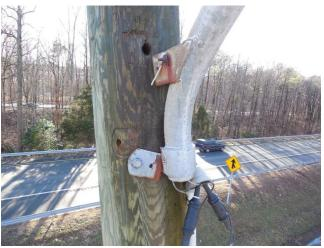
Photo 6.59 Chord to timber pole connection plate cracked, bolt missing, wiring exposed
