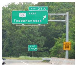
Photo 1.29 Cantilever, two chord plane truss
