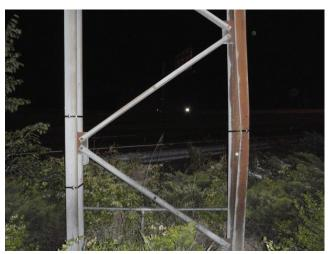
Photo 3.20 Out of plane distortion
