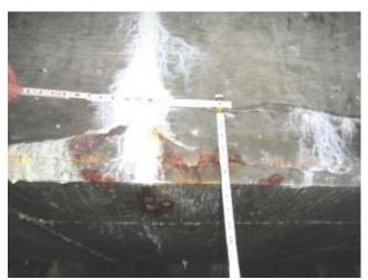
Photo 3.5 Cracking with exudation and rust straining
