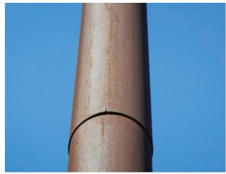
Photo 3.31 Crack at high mast light pole slip joint
