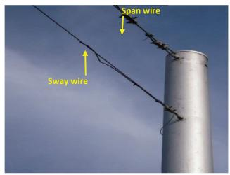
Photo 1.55 Span/Sway wire to pole attachment
