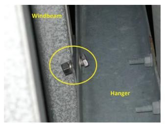
Photo 4.83 Misaligned and loose bolt at windbeam to hanger connection
