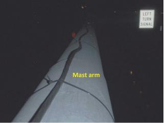
Photo 5.71 Improperly secured cable fastened to top of mast arm
