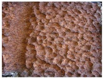
Photo 3.18 Corrosion with heavy pitting and section loss
