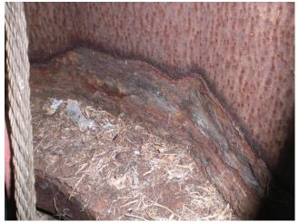
Photo 3.29 Corrosion with section loss
