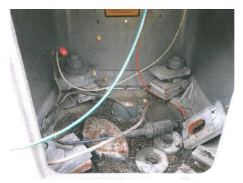
Photo 6.36 Improperly sized, incorrect, and excess washers
