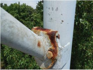
Photo 6.57 Chord to pole connection corrosion
