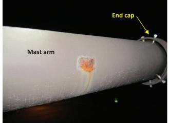
Photo 5.64 Area of corrosion on mast arm
