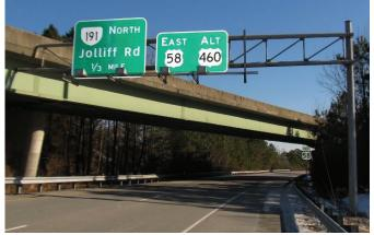
Photo 1.28 Overhead span with fixed attachment
