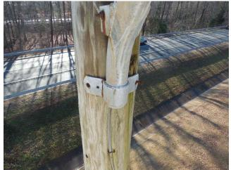
**Photo 6.58** Chord to timber pole missing and loose lag bolts
