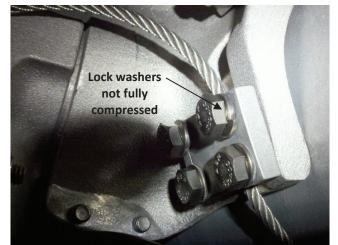
**Photo 5.86** Loose bolts at cable clamping connection to orbital bracket
