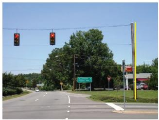
Photo 5.40 Out of plumb pole, note welded splice in pole near mid-height
