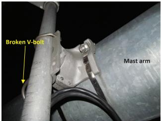
**Photo 5.84** 1 of 2 V-bolts broken at gusseted tube connection to orbital bracket
