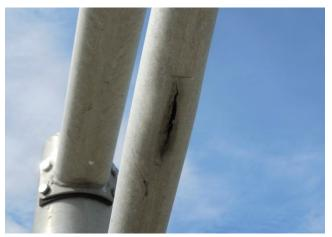
Photo 6.62 Lower chord cracked/ruptured along bottom
