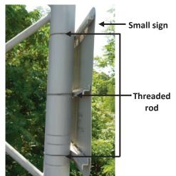
Photo 1.20 Attachment to vertical support, straps
