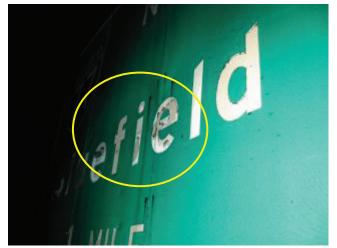
Photo 4.90 Peeling/Delamination of lettering on sign panel
