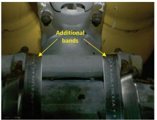
**Photo 5.87** Additional stainless steel bands installed at orbital bracket
