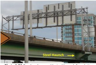
Photo 1.26 Overhead span with steel haunch foundation
