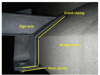
**Photo 1.42** Attachment to bridge beam, saddle clamp, front view
