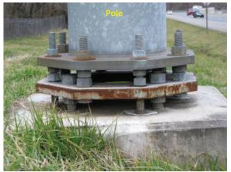
Photo 4.46 4-bolt pedestal to 8-bolt base plate retrofit
