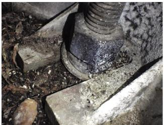
Photo 6.37 Improperly sized washer embedded into slot
