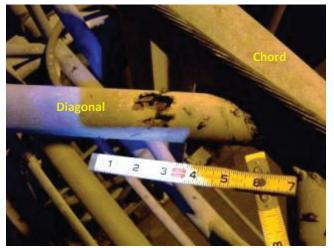
**Photo 4.53** Area of 100% section loss in upper diagonal member of chord truss
