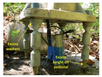
**Photo 6.29** Coupler with excess washers and excess height off pedestal
