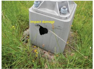
Photo 6.34 Transformer base with impact damage
