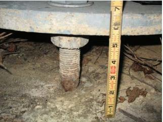
**Photo 4.27** Excessive top of pedestal to bottom of base plate height
