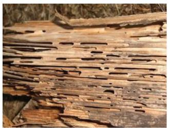
Photo 3.14 Insect damage (carpenter ant)
