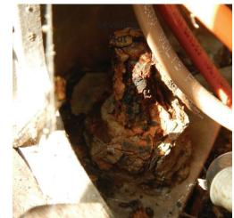
**Photo 6.22** Heavy corrosion and section loss to anchor bolt and nut inside transformer base
