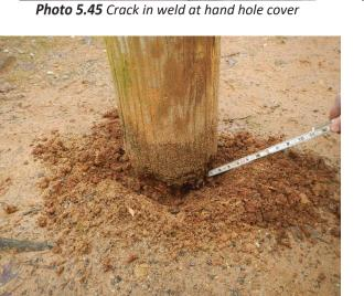
Photo 5.47 Timber pole decay below grade
