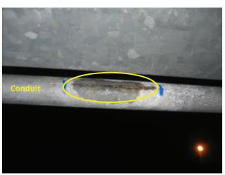
Photo 4.97 Cracked conduit member
