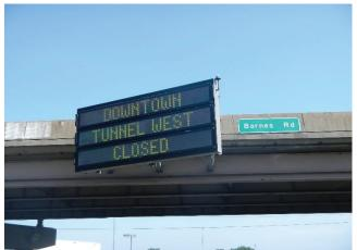
Photo 1.39 Bridge parapet mount VMS
