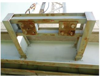
**Photo 5.21** Corrosion of steel haunch (Sign structure shown for illustrative purposes only)
