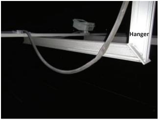
**Photo 4.100** Loose conduit hanging below hangers and reducing vertical clearance
