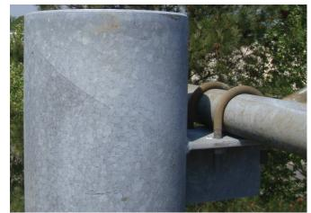
Photo 1.14 Simple truss support, seated on chair
