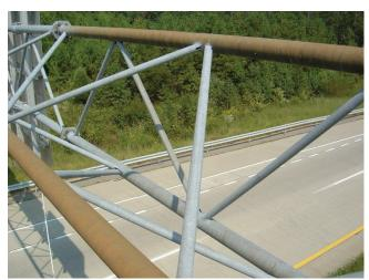
Photo 3.24 Coating failure of galvanizing
