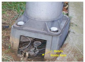
Photo 6.32 Transformer base filled with debris
