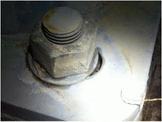
Photo 4.29 Oversized base plate hole and inadequately sized flat washer under top nut
