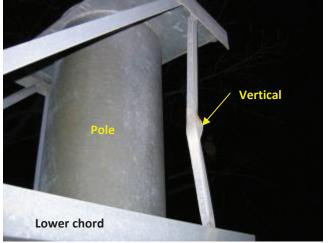
Photo 4.57 Bent vertical truss at end of chord box truss
