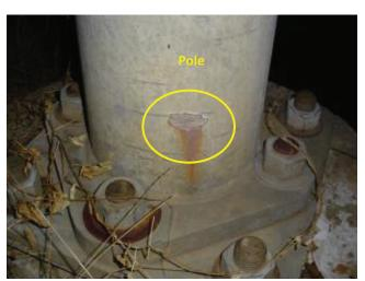
**Photo 4.39** Minor impact damage/dent in pole with damaged galvanizing and corrosion
