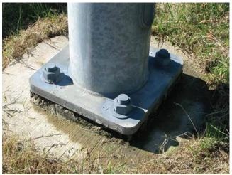
Photo 4.21 Deteriorated grout pad with moisture leakage
