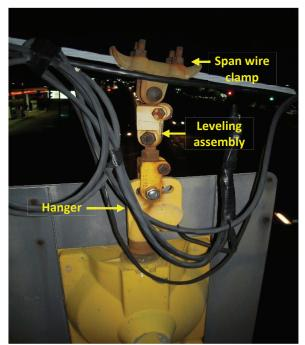
Photo 1.52 Span wire clamp
