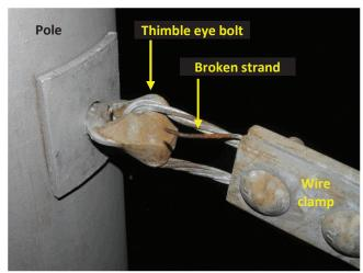
Photo 1.54 Span wire to pole attachment
