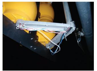
Photo 5.99 Loose wires at bottom of signal head
