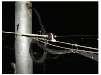
Photo 5.61 Line attached to span wire at span wire to pole connection
