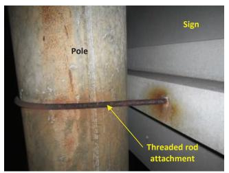
*Photo 4.48 Corroded sign to pole connection hardware*
