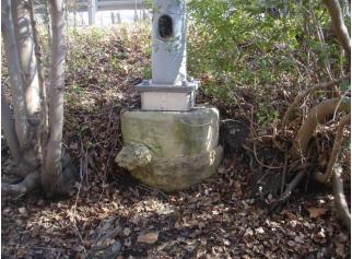
**Photo 6.11** Erosion of pedestal, note hand hole cover missing
