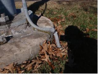
Photo 5.19 Damaged conduit at pedestal
