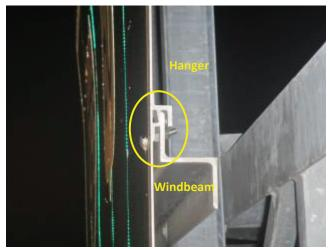
Photo 4.88 Misaligned sign panel to windbeam through bolt
