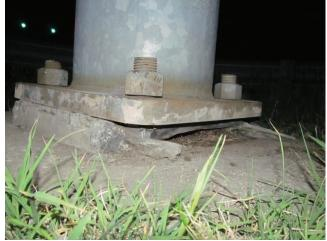
Photo 5.23 Deteriorated grout pad with exposed anchor bolts
