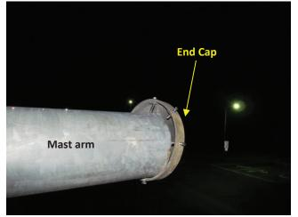
**Photo 5.72** Improperly sized and fastened end cap at end of mast arm
