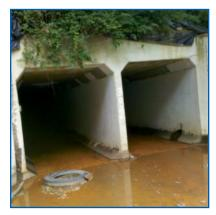
Presence of iron bacteria in culvert, as well as in stream Note the orange-brown color
