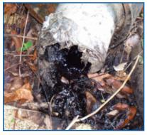
"Close up" of discharge of oily substance from pipe
