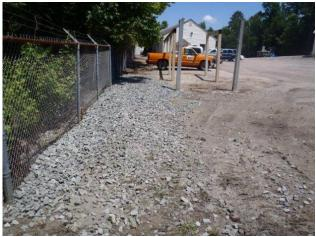
Rock Aprons to control fines in areas of sheet flow drainage discharge areas
