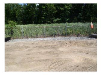
Silt fencing and rock aprons at sheet flow discharge areas on stone lots
