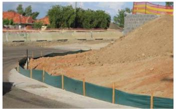
Silt Fence around soil pile
