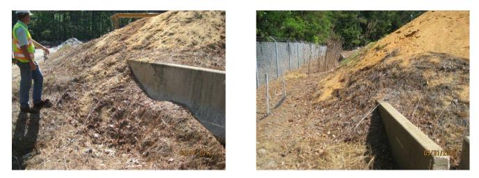
Clean up of sand/erodible materials pushed overtop of jersey-wall control structures
