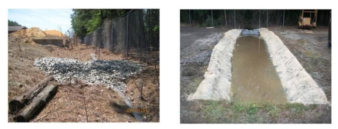
Rock Check Dams and Drainage Ditch Soil Stabilization
