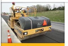
I-81 project recycles pavement To rebuild part of Interstate 81 in Augusta County, VDOT is using three innovative paving processes that will reduce construction time by two-thirds, save millions of dollars and recycle existing materials back into the new pavement. The "in-place pavement recycling" project employs full-depth reclamation to rebuild the underlying structure plus cold-in-place recycling and cold central-plant recycling for the first time together on a U.S. project.
