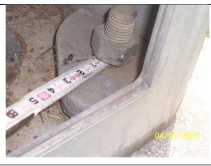
Loose anchor bolt nut at luminaire base
