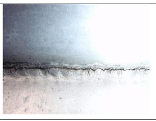
Crack in luminaire bracket saddle to connection plate weld
