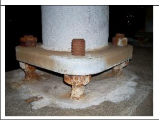
Rusted anchor bolts and missing nut
