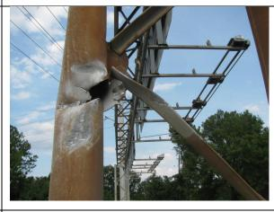
Column torn and bent 3" at point of impact
