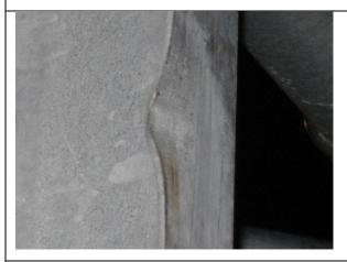
Damaged & bent flange of vertical hanger
