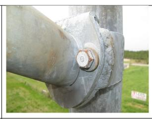
Weld around upper chord to mounting plate connection 50% complete
