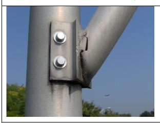
Fracture in weld of lower arm tube to luminaire pole connection
