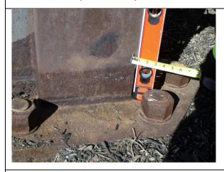
Section loss to the bottom of the pole.
