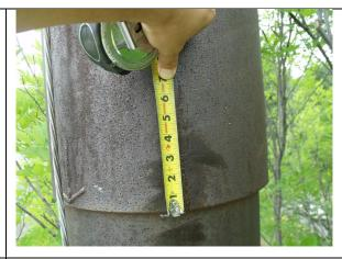
4" vertical crack at the slip joint
