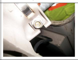
Nut on strap bolt for signal from pole lacks 50% thread contact
