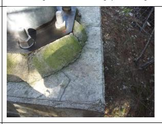
Deteriorated and cracked grout
