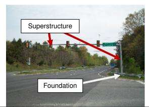
Figure 7 – Cantilevered Arm Traffic Signal Structure
