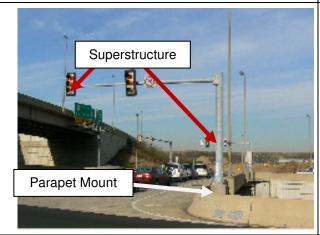
Figure 9 – Parapet Mount - Traffic Signal Structure
