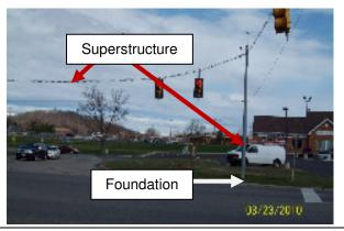
Figure 8– Span Wire Traffic Signal Structure
