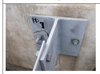
Failed bolt (circled) at parapet mount.
