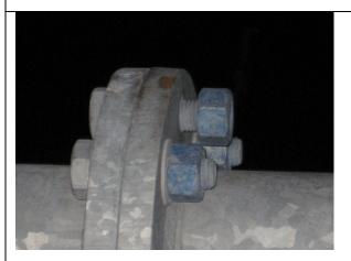
Loose Bolt at splice plate.
