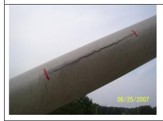
6" crack in lower chord of luminaire
