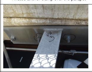
Two failed bolts (circled) at parapet mount
