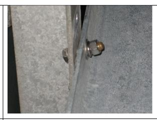
Poor vertical hanger connection with the Z-bar
