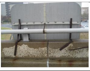
Twisted anchor clamp over the parapet
