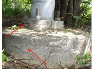
Deteriorated grout pad and cracked pedestal
