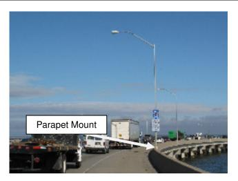
Figure 6 – Parapet Mounted Luminaire Structure
