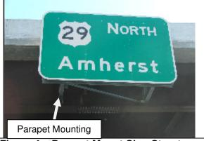
Figure 4 – Parapet Mount Sign Structure
