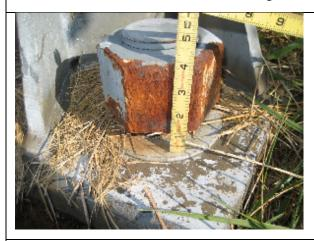
Loose anchor bolt with 1" gap between nut and base plate
