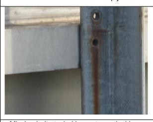
Missing bolt at wind beam to vertical hanger connection
