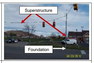
**Span Wire Traffic Signal Structure**
