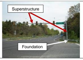
Cantilevered Mast Arm Traffic Signal Structure
