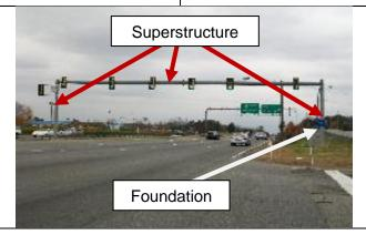
**Overhead Span Traffic Signal Structure**
