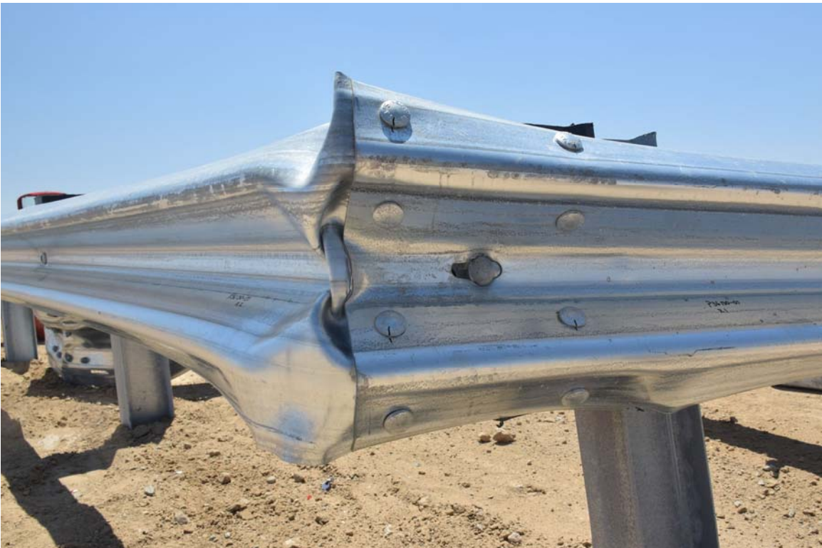
FIGURE 36. Test Article Damage
