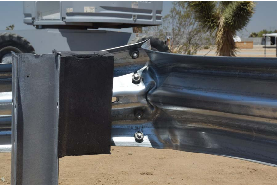
FIGURE 38. Test Article Damage
