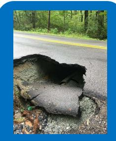
Figure 1: Roadway Closure as a Result of a Flooding Event
