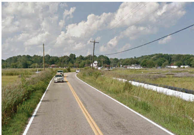
Wythe Creek Road looking northbound from Hampton at the existing bridge and causeway.
