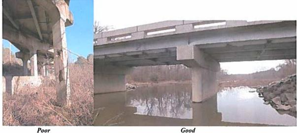
Figure 11: Comparison of Bridges in Poor and Good Conditions
