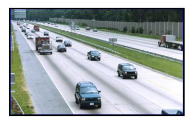
Concrete noise walls take less space than earth berms. Many attempts are being made to construct noise barriers that are visually pleasing and that blend in with their surroundings.
